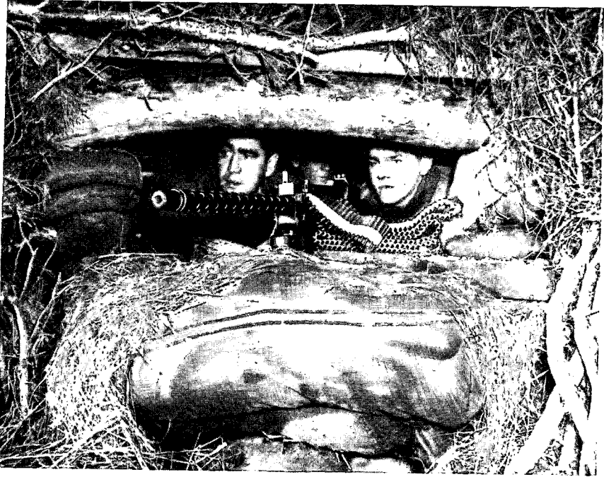
Figure 81. Machine gun emplacement using logs to support natural camouflage.
