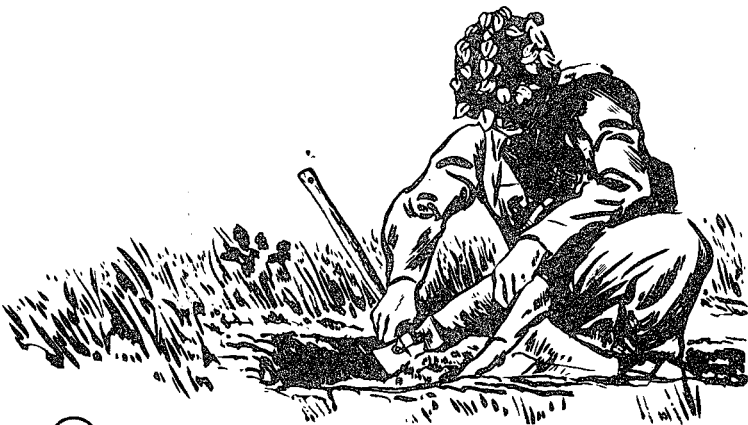
② SPOIL BEING REMOVED CORRECTLY
