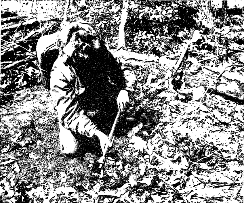
Figure 67. Removing natural camouflage material before construction of position.
