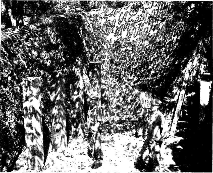
Figure 69. Work being done on bunker, using net to conceal activity.
