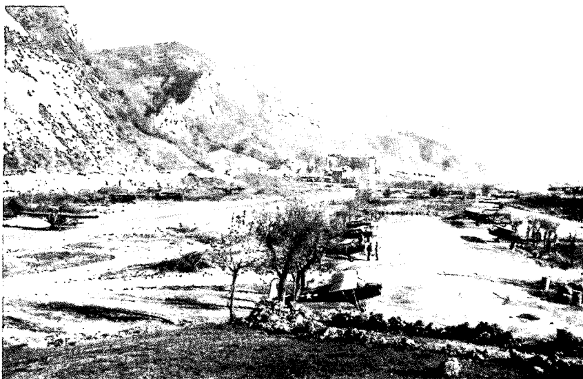
Figure 166. Hasty airfield built during World War II.
